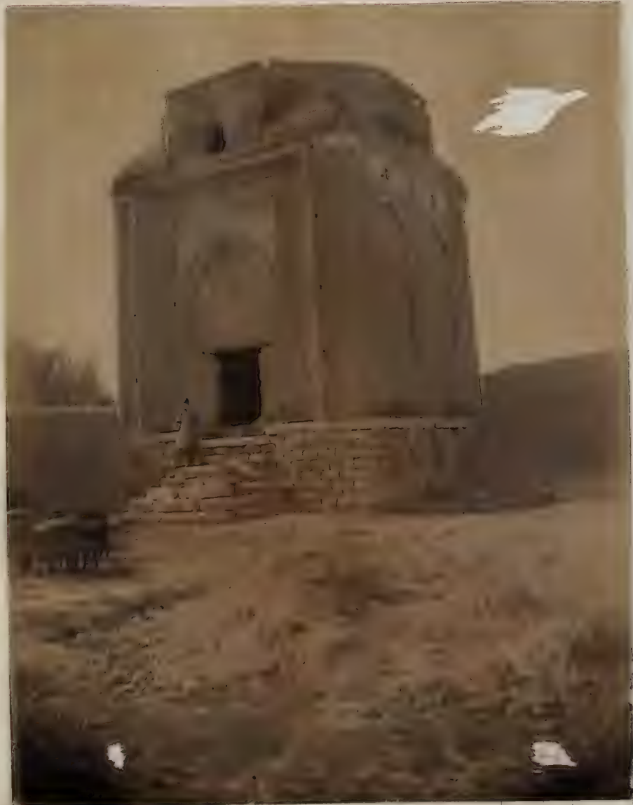
Tower at Baragha
